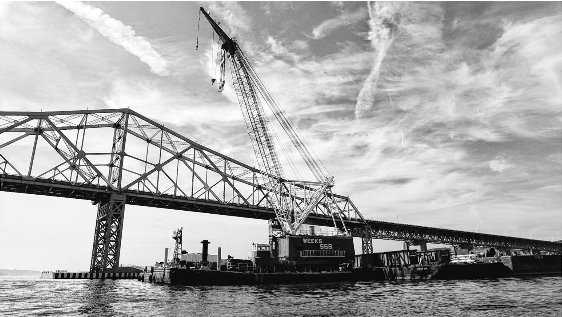
Construction barges carrying cranes and other heavy equipment are visible Oct. 3 as work progresses in the construction of the new Tappan Zee Bridge. The work includes dredging for platforms and the driving of pilings. JOE LARESE/THE JOURNAL NEWS
