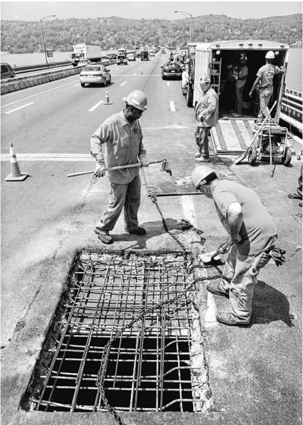
Thruway workers get ready to place a large steel plate over a hole on the deck of the Tappan Zee Bridge on June 1, 2005. A hole, three feet around, broke through the deck the day before; the crew cleaned the area, placed new rebar on top and filled the hole after rush-hour traffic. JOURNAL NEWS FILE PHOTO
